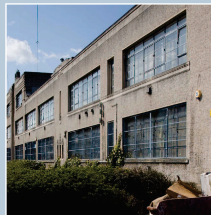
Former Niddrie Marischal School, Edinburgh. Designed in Art Deco style in 1935 by architects Reid & Forbes. The strips of blue-painted steel windows have two opening methods: horizontal pivots and small hoppers. The ground-floor windows are protected from vandalism by discreet metal mesh screens painted in the same colour. © N. Haynes.
