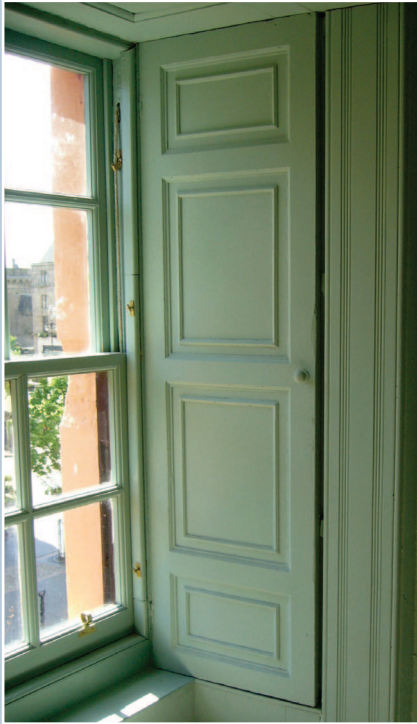
Associated fixtures such as traditional timber shutters contribute to the interest and character of a window.
