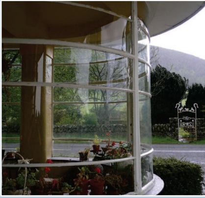
A distinctive, metal framed bay window at the Crook Inn, Tweedsmuir, Peeblesshire.
