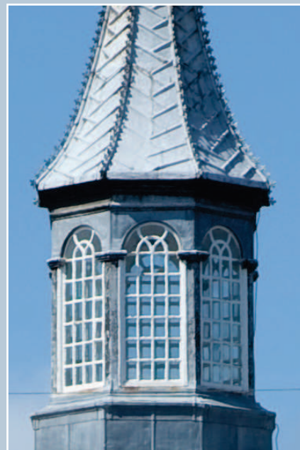
Fixed small-pane windows in the cupola of Robert Gordon's Hospital, Aberdeen, designed by William Adam in 1731–32. Thick astragals (glazing bars) and small panes of glass are typical of this period of design.
