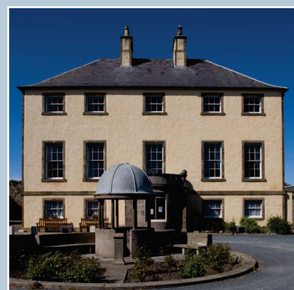
Banff Castle, Aberdeenshire. Here the size of the windows at the first floor indicate that this was the principal storey where the public rooms were located. The symmetrical arrangement and careful proportioning of the windows is the main architectural feature of the building. © N. Haynes.
