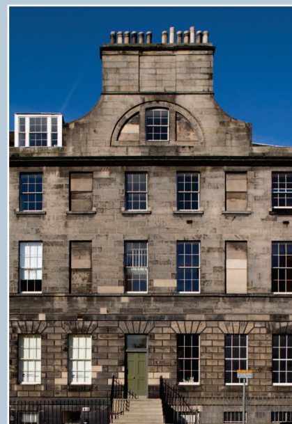
South Charlotte Street, Edinburgh. The blind openings are detailed with sills and a 'meeting rail' to maintain the symmetry of the architectural elevation. The chimney flues pass behind the blind windows. © N. Haynes.
