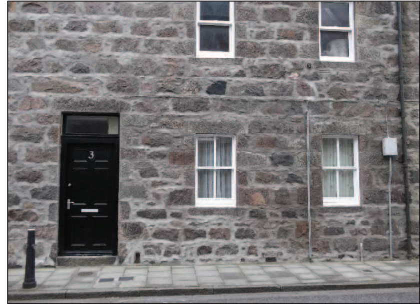
Replacement windows will generally require to be white
