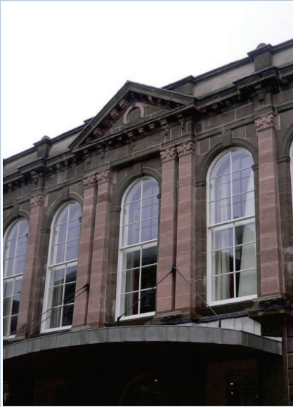
Webster Theatre, Arbroath. Large clear sheets of internal secondary glazing were installed here during recent refurbishment.
