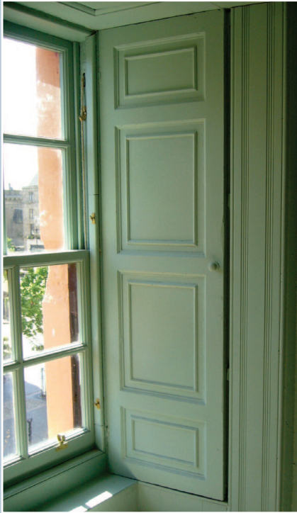
Associated fixtures such as traditional timber shutters contribute to the interest and character of a window.
