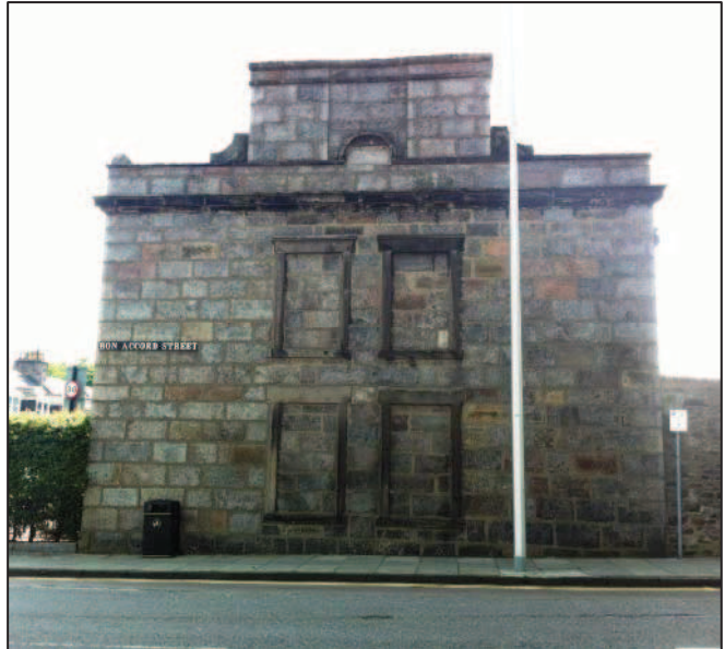
Example of blocked up windows in Ferryhill
