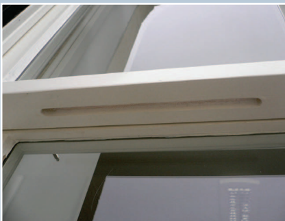
A view of the underside of the meeting rail of a new timber sash and case window at Castlemilk Stables, Glasgow. A discreet slot ventilator in the meeting rail allows ventilation without the need for obtrusive external fixtures.
